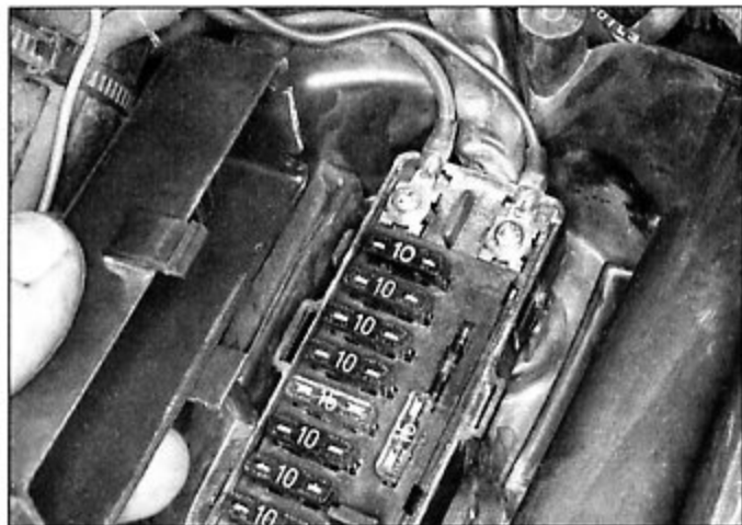
5.1b . . . spare fuses are stored in the fuse block
