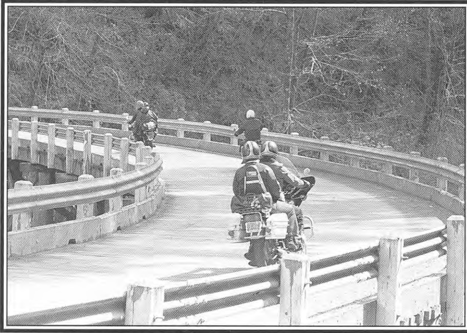
This wooden bridge deck is treacherous in the rain.
