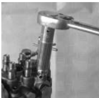
Remove the joint, (FO inlet pipe).
