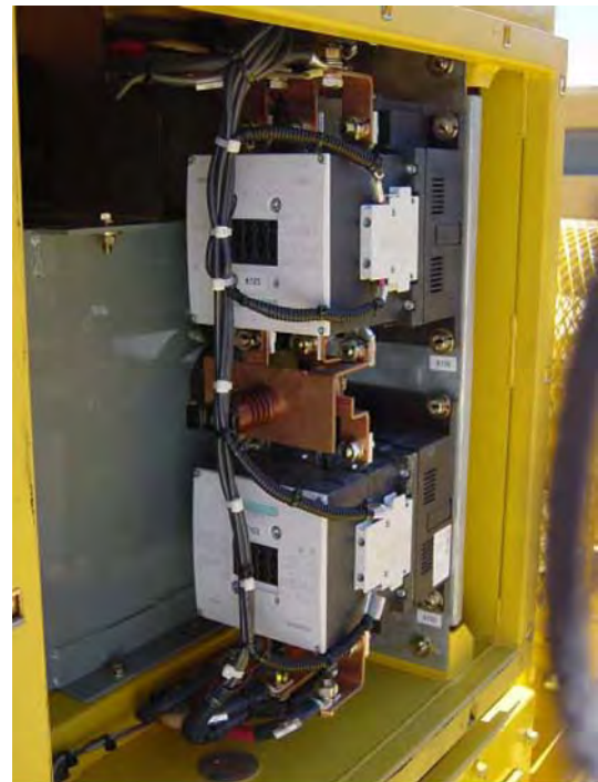
FIGURE 10-44. CONTACTORS K105 AND K103, FRONT VIEW (LOCATED ON REAR SIDE OF CONTROL CABINET IN UPPER RIGHT DOOR)
