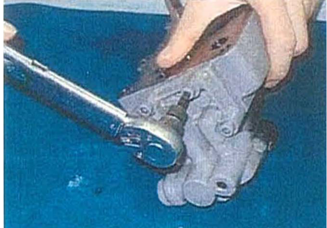
Installing valve casing (325)
