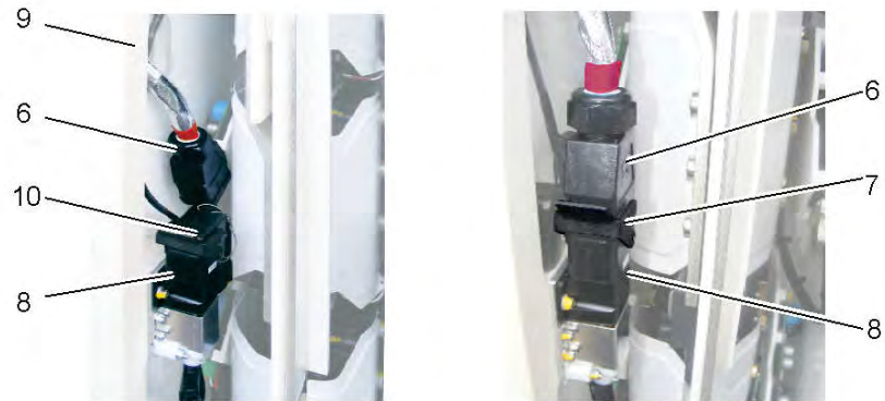
Fig. .8-322: Connect the control connections
