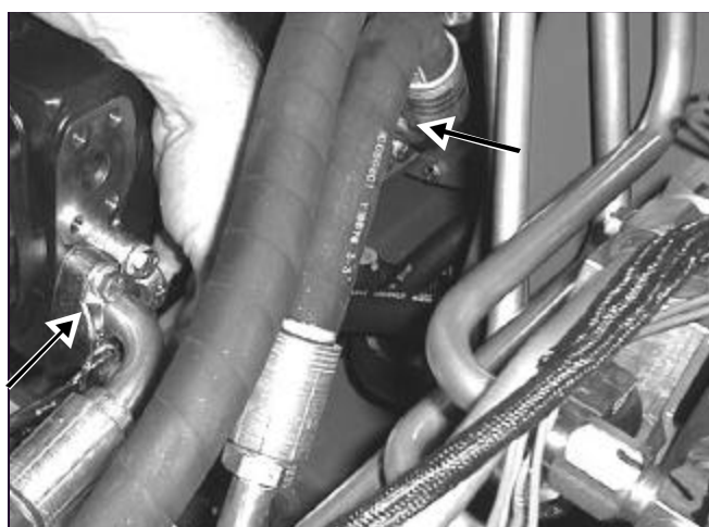
Fig. 7-13 Hoses to remove off hydrostatic pump for pump removal. There is a second set of these hoses on pump closer to engine.
