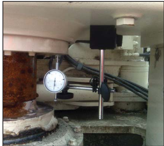
Fig. 6-15 Main Shaft Bearing Preload checking
