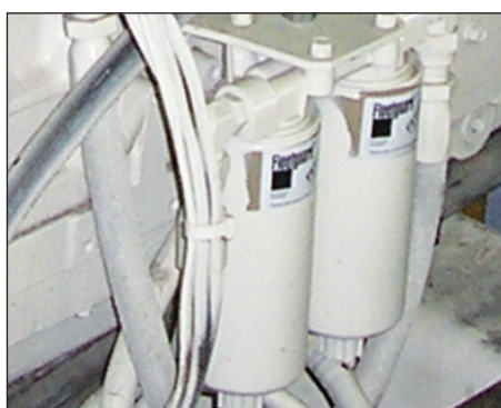
Cummins QST30 Fuel Filter (2)
