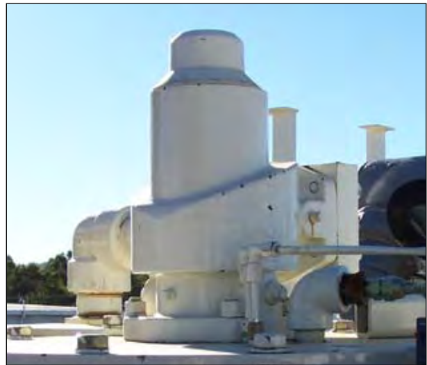
Minimum Pressure Valve
