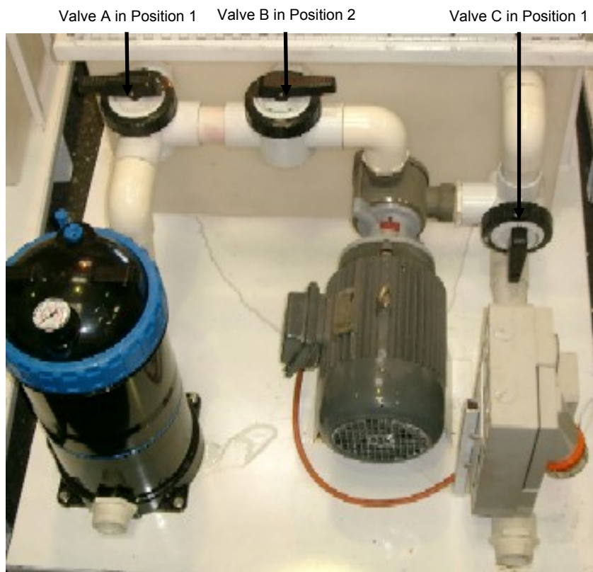
TURBO WASH VALVE POSITIONS—EMPTYING
