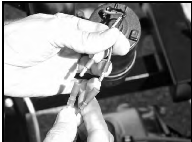
Figure 11c-48 Bed Lift Motor Wires
