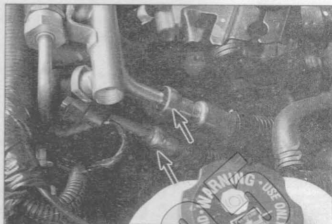
4.7b Location of the inlet and return lines (arrows) on the fuel rail
