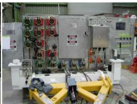
Transformer station front view
