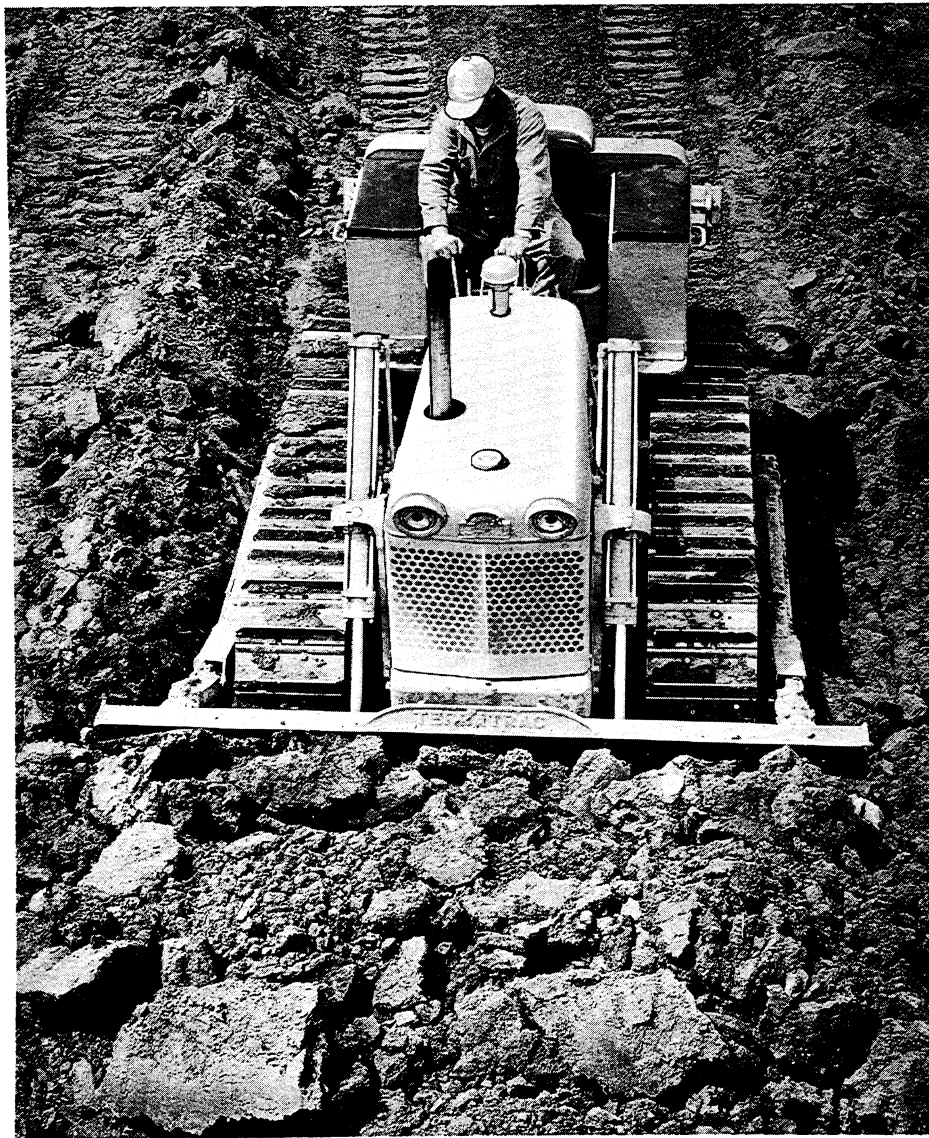
1000 Bulldozer Cutting A Trench
