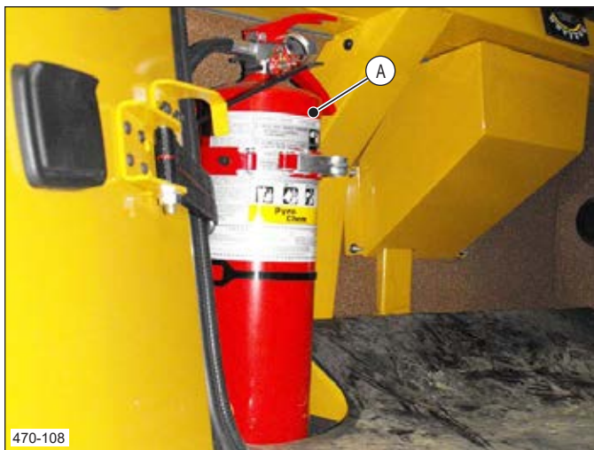
A Portable Fire Extinguisher
