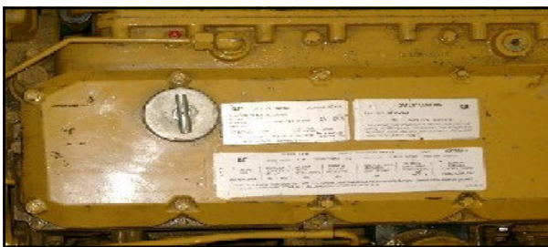
Figure 5.2.3 Engine fill point
