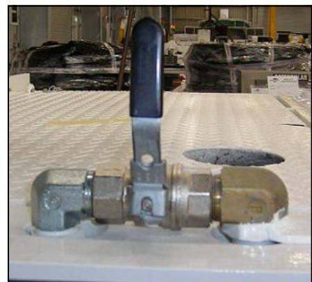
Figure 5.2.2- Main Air Isolating Valve
