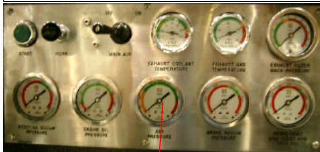
Figure 4.1.1 Air pressure isolation and indication in operators compartment
