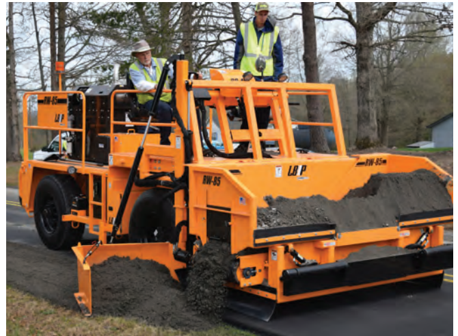
Figure 4-42. Road Shoulder Work with the RW85 Road Widener
