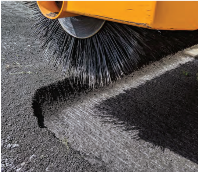
Figure 4-13. Sweeping Mill Cut Road Construction
