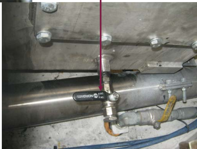
Low Water Shutdown Test Ball Valve
