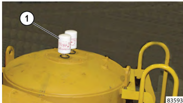
Figure 7-1 HYDRAULIC TANK SERVICE
