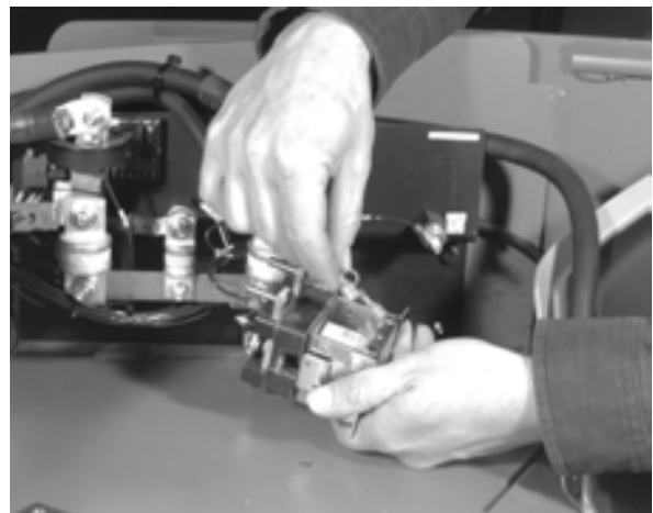
Figure 5-47: Disconnect Wires from Terminals
