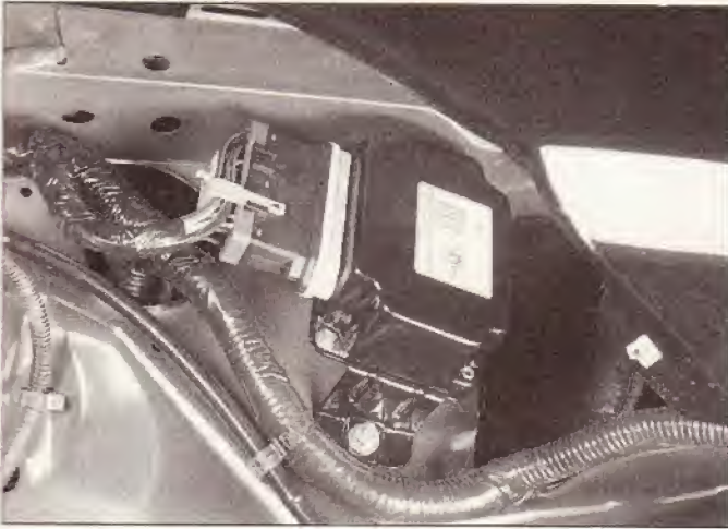
3.3a Remove the center bolt, disconnect the CCRM harness connector and check for battery voltage on terminal number 11 with the ignition key ON (engine not running). This checks power from the 20 amp fuel pump fuse
